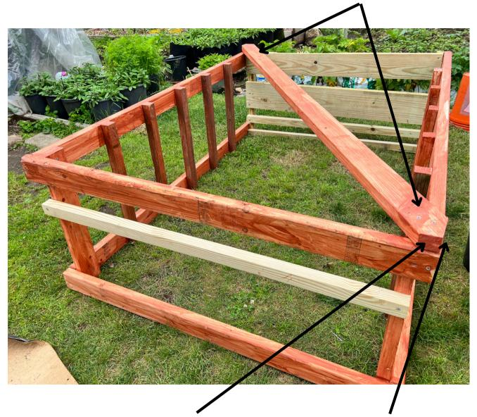
Cut off any excess wood on both sides
