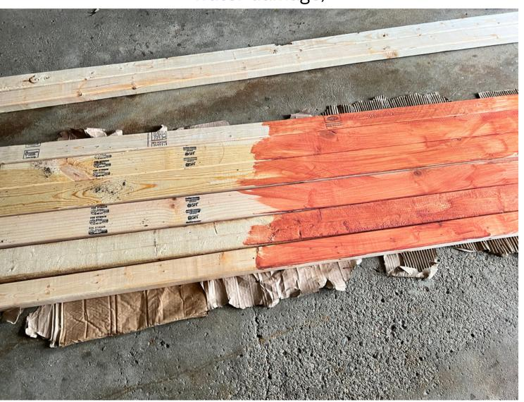
I recommend doing at least 2 or 3 coats to protect the wood. Make sure all surfaces are covered even the ends.
